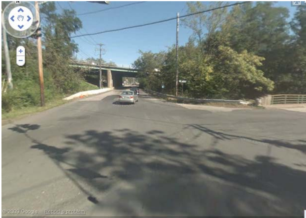
SOUTH PASCACK ROAD AT GARDEN STATE PARKWAY NORTHBOUND OFF-RAMP/OLD NYACK TURNPIKE, LOOKING NORTH
