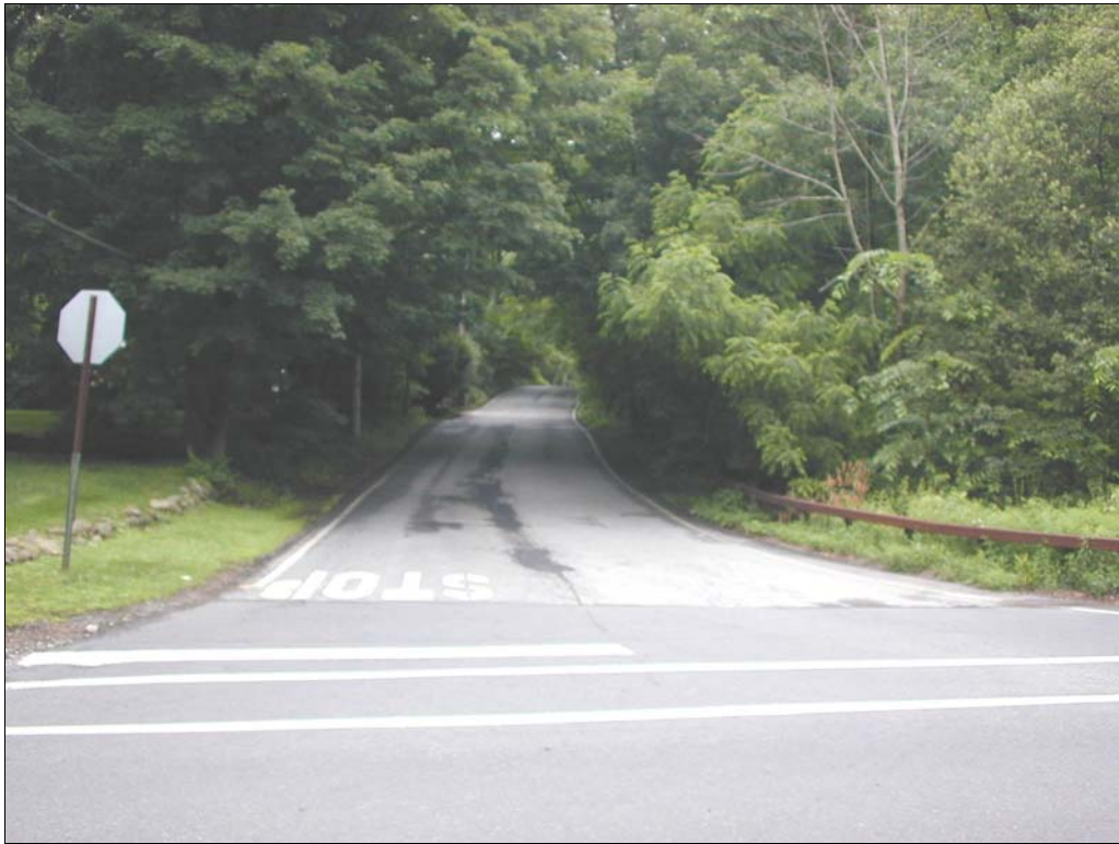
WILLIAMS ROAD AT SOUTH PASCACK ROAD, LOOKING WEST
