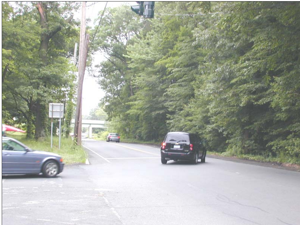
RED SCHOOLHOUSE ROAD AT GARDEN STATE PARKWAY SOUTHBOUND OFF-RAMP, LOOKING SOUTH
