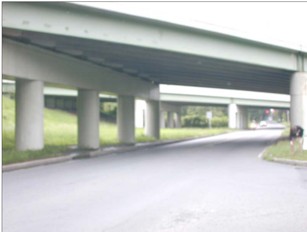
RED SCHOOLHOUSE ROAD AT GARDEN STATE PARKWAY NORTHBOUND ON-RAMP, LOOKING NORTH
