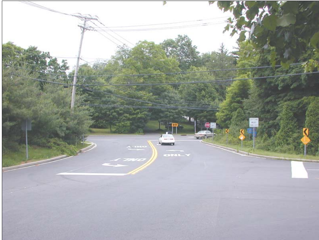
SCOTLAND HILL ROAD AT SOUTH PASCACK ROAD, LOOKING EAST
