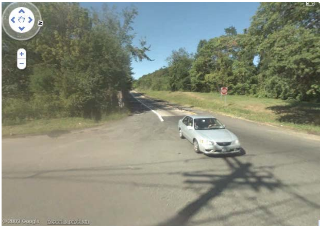
GARDEN STATE PARKWAY NORTHBOUND OFF-RAMP AT SOUTH PASCACK ROAD, LOOKING WEST
