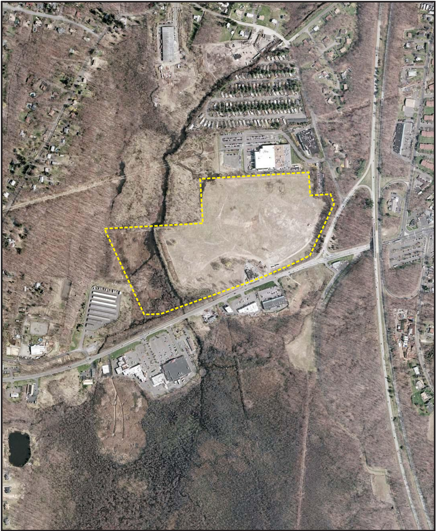
Figure 3.3-1: Aerial View of the Project Site Minisceongo Park
