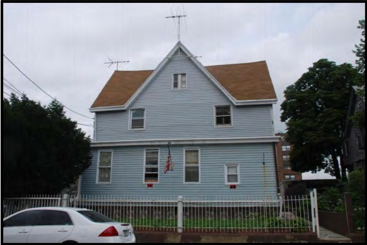
Photo 8: 65 Buena Vista Avenue. View west..
