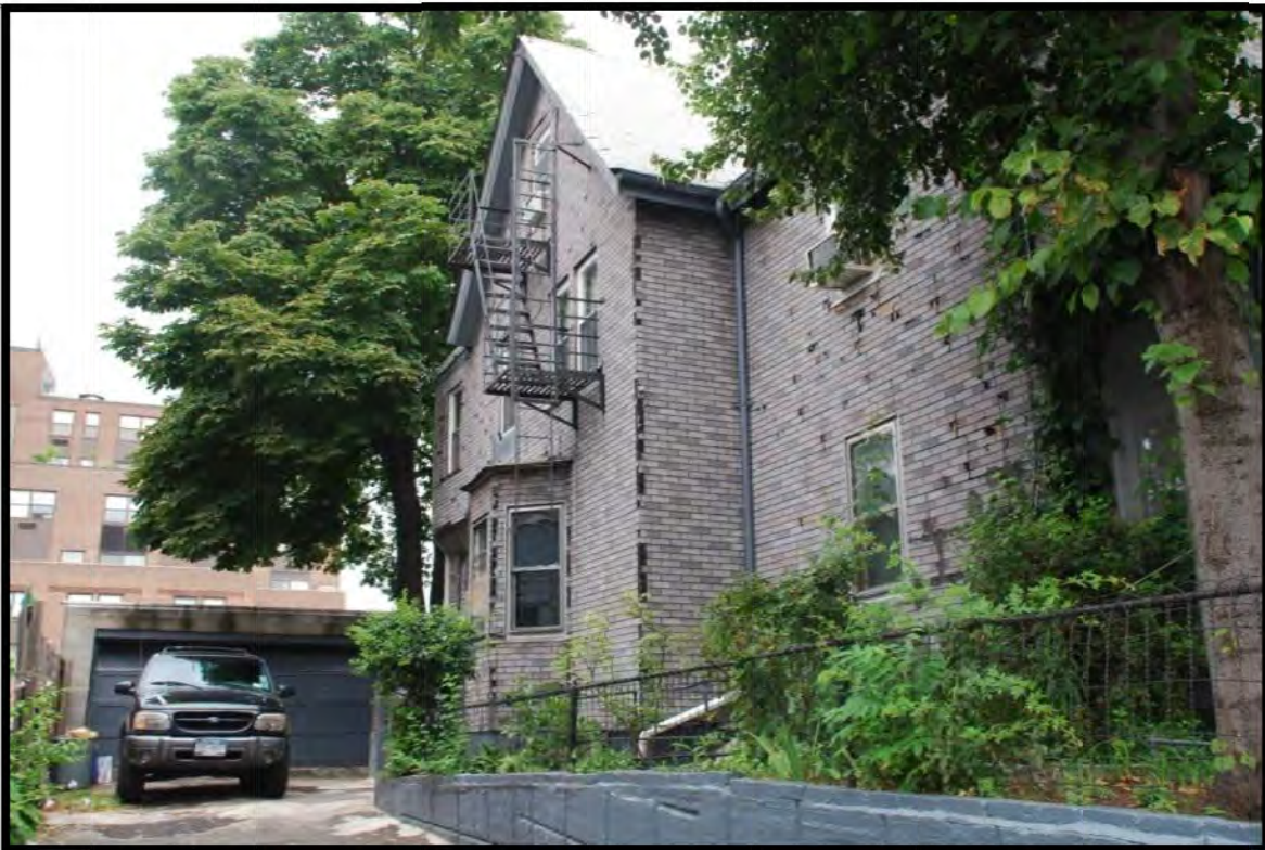
Photo 7: 61 Buena Vista Avenue. View to northwest.
