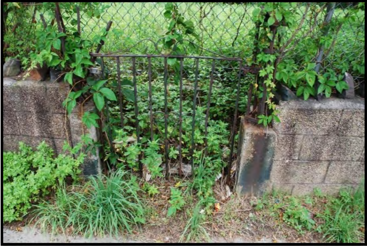
Photo 17: Wrought iron gate and break in cinder block wall indicates entrance to house formerly located at 56 Buena Vista Avenue. View to northeast.
