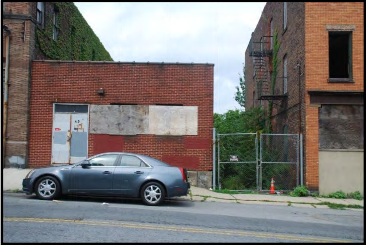
Photo 2: 43-45 Buena Vista Avenue. One-storey brick commercial building with alleyway to north. View to west.
