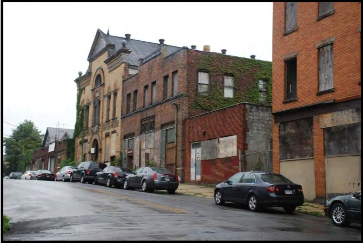
Photo 37: View of Teutonia Hall from southeast
