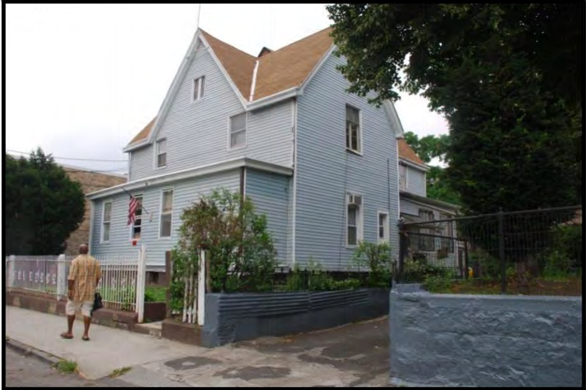
Photo 9: 65 Buena Vista Avenue. View to southwest.
