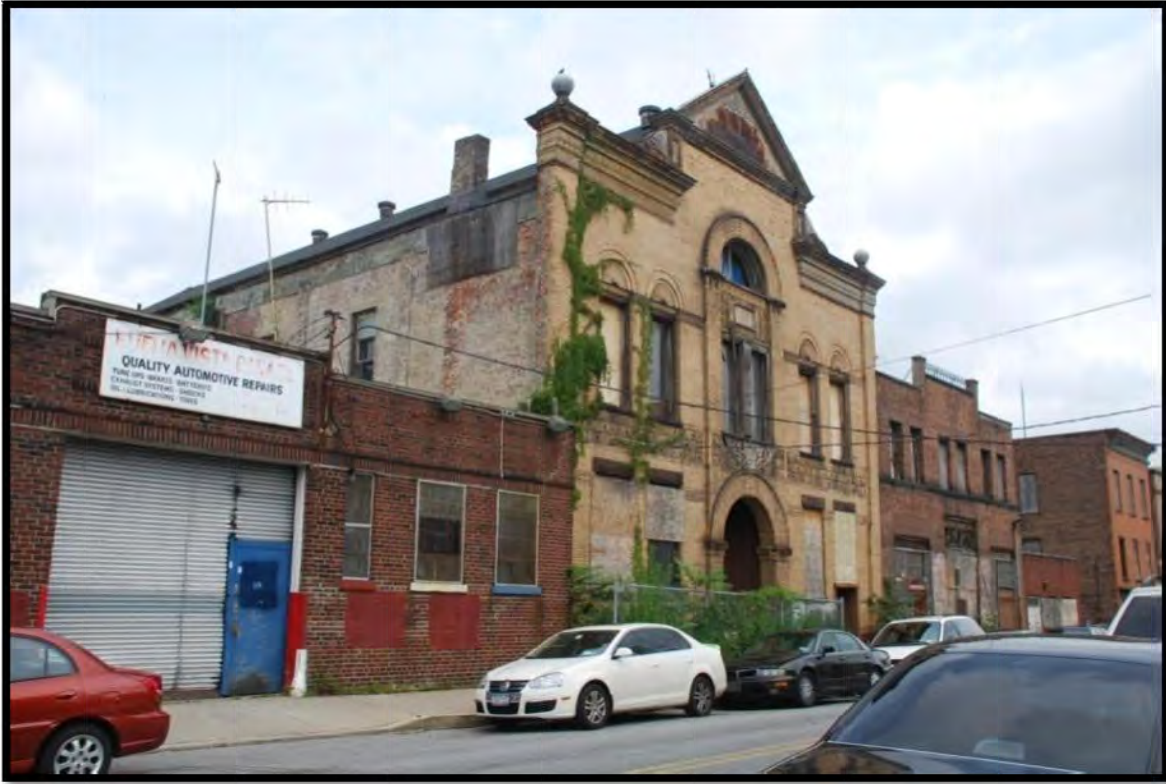
Photo 4: 49-51 Buena Vista Avenue (Teutonia Hall). View to northwest.
