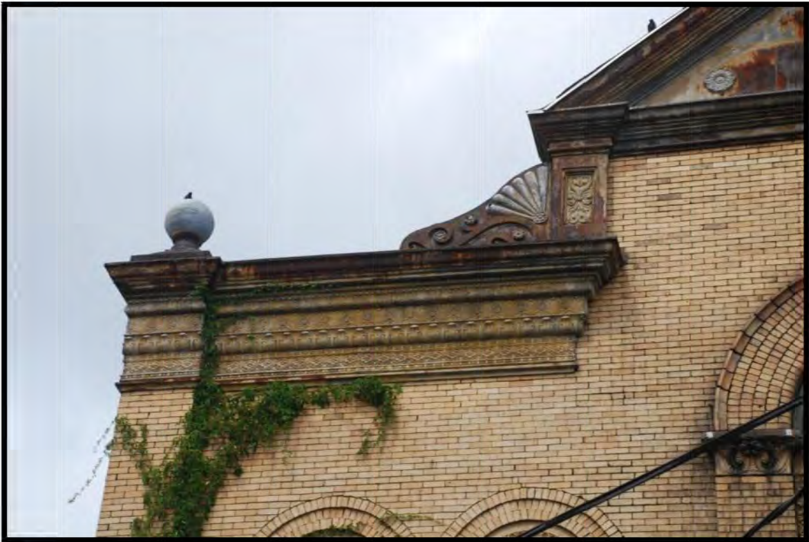
Photo 30: Roofline on southern part of Teutonia Hall included ball finial and sunburst. View to southwest.
