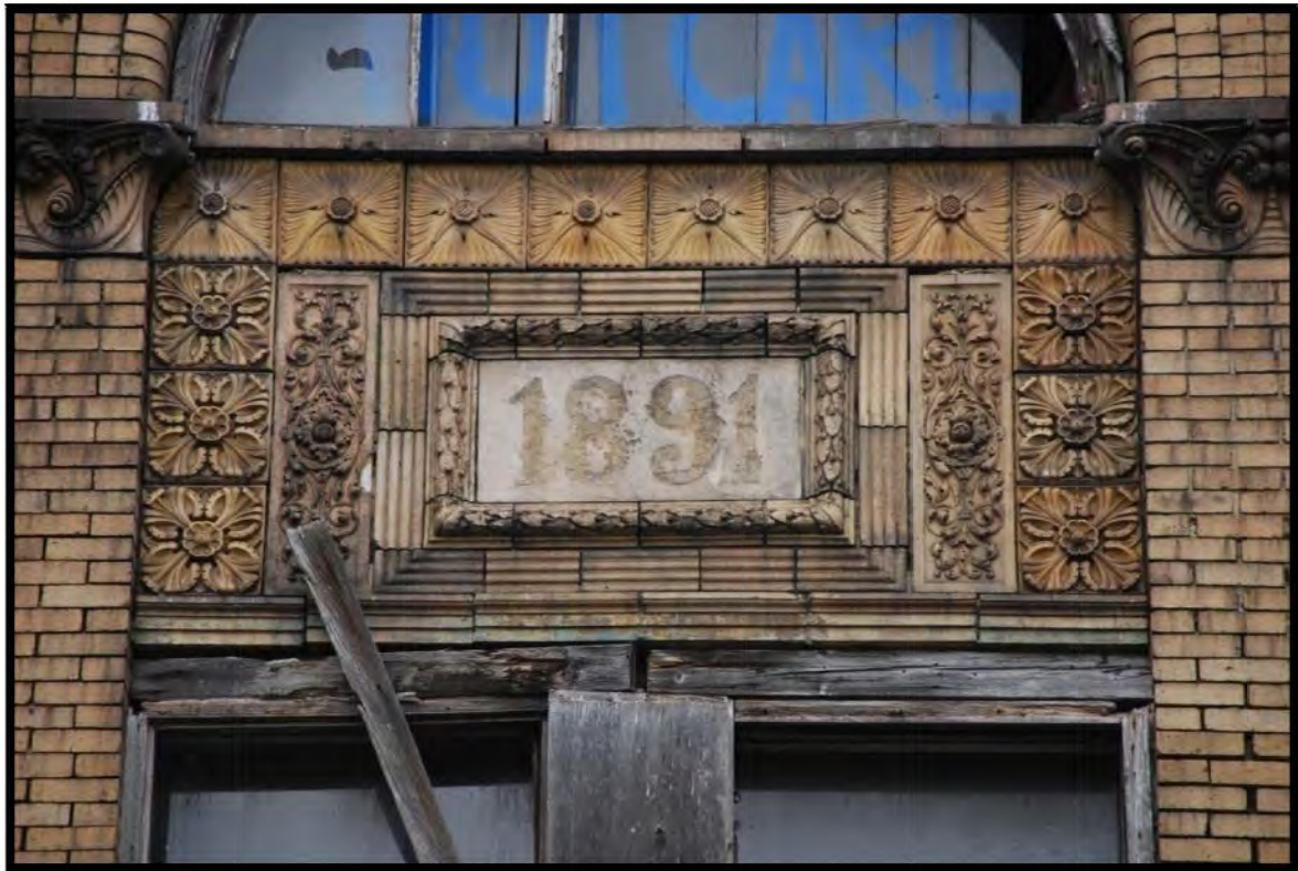
Photo 29: Date in upper center window of Teutonia Hall. View to west.
