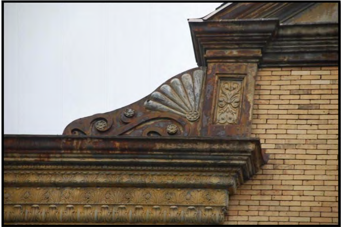
Photo 31: Detail of pediment and corner detail on façade roofline of Teutonia Hall. View to east.
