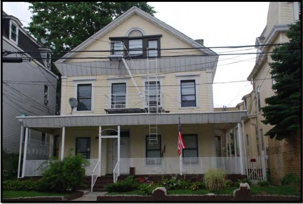
Photo 12: 68 Buena Vista Avenue. View east.
